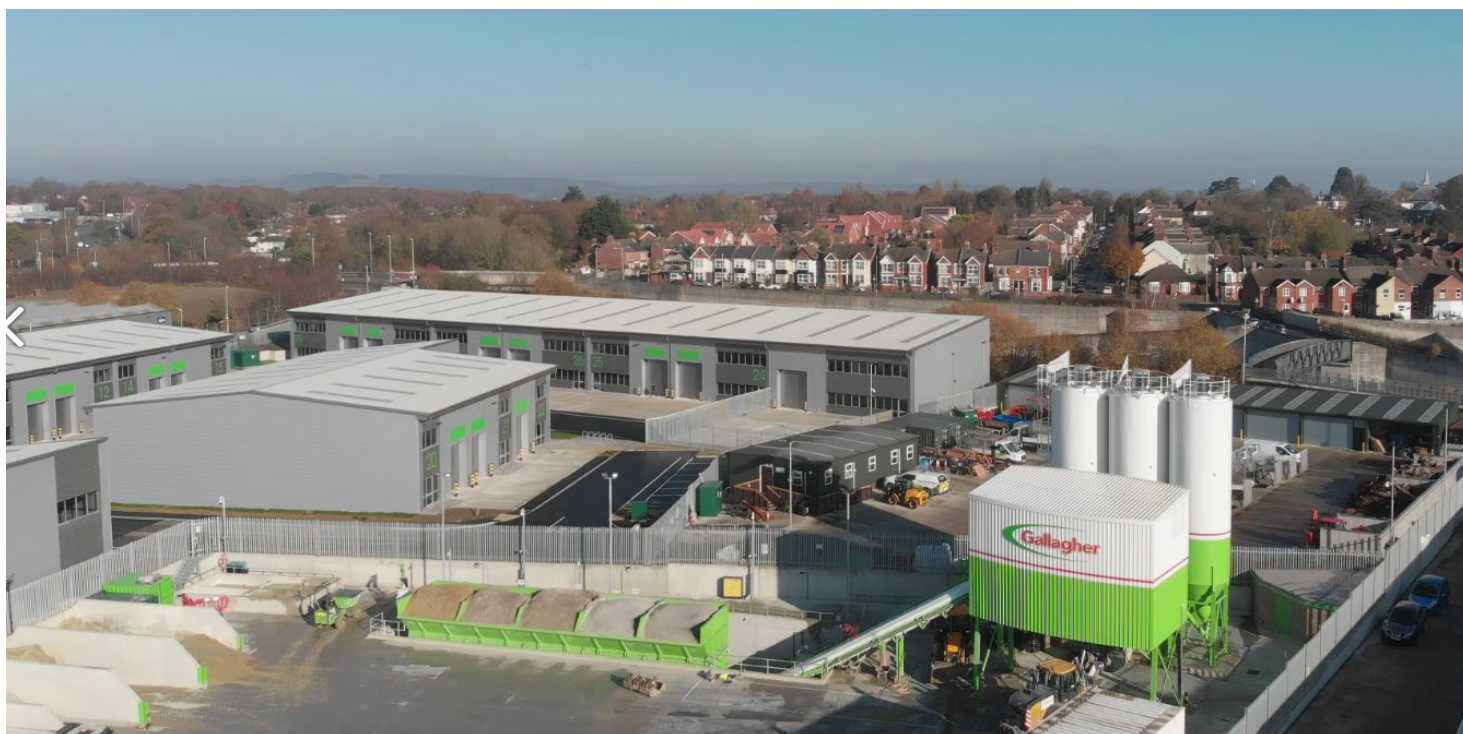
Figure 4: Plot 3 Industrial units as completed.
